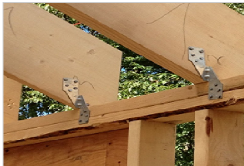
Hurricane clips on roof trusses
