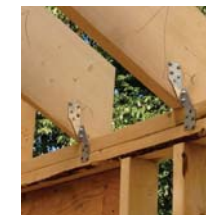
Fig. 8. Hurricane clips on roof trusses. Photo Credit: Buildipedia
